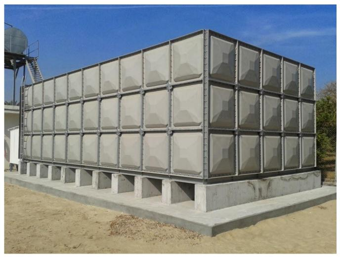
GRP HOT – PRESSED SECTIONAL WATER TANKS.
